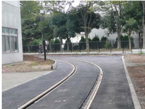
Full Scale LRT Test Track
